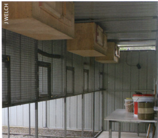
Suspended aviaries are a popular design due to the birds' reduced access to debris and associated pathogens and ease of cleaning
