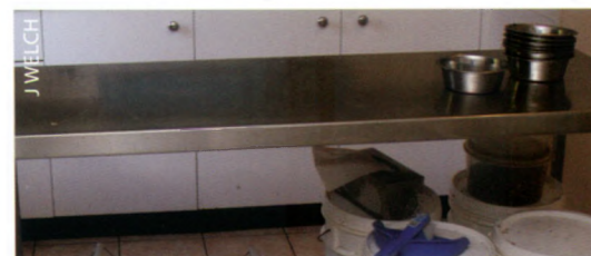
A stainless steel bench provides an efficient and hygienic food preparation area
