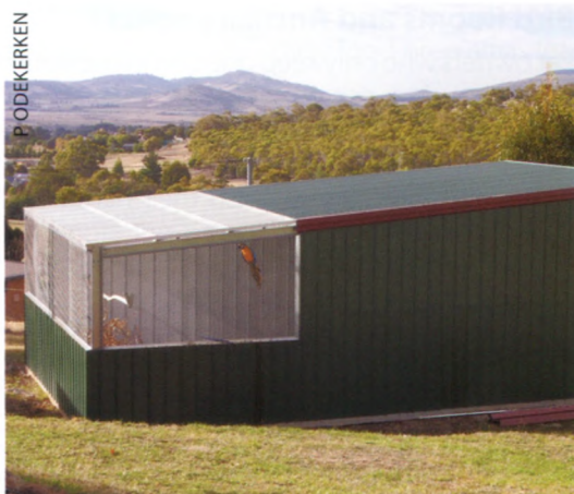
This aviary design has incorporated extensive predator and rodent protection, as well as shelter from a windy and cold climate
